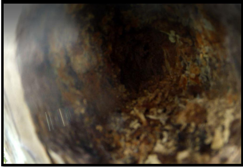
Photo 29: Potential Roost 4 Cavity
