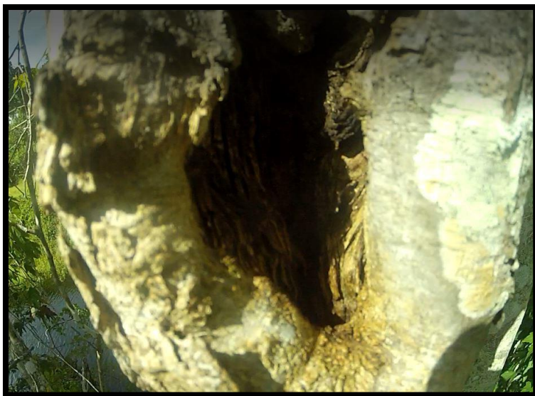
Photo 23: Potential Roost 1 Cavity
