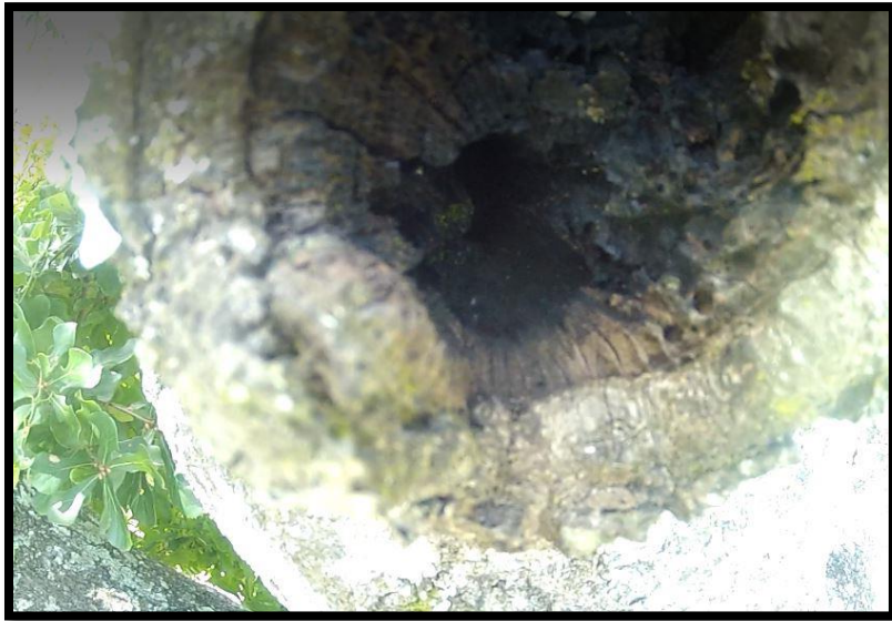
Photo 27: Potential Roost 3 Cavity
