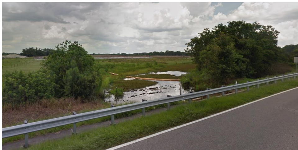
Partin Canal - Major Cross 1 Looking NE
