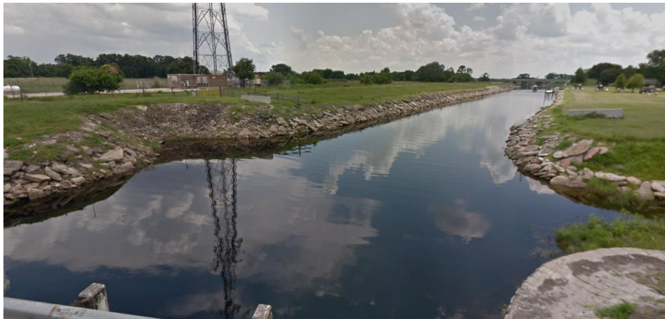
Canal C-31 – Looking SW from Highway Bridge Structure
