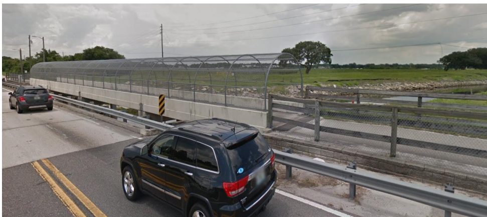
Canal C-31 – Looking N from Highway Bridge Structure at Pedestrian Bridge Structure
