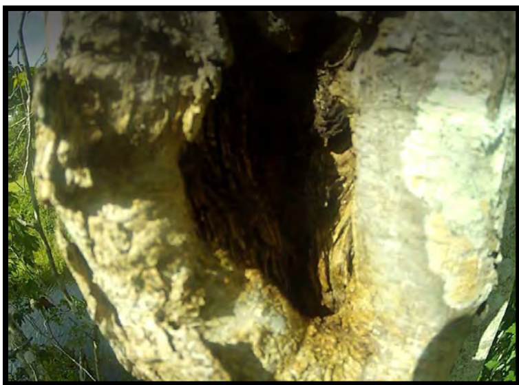
Photo 23: Potential Roost 1 Cavity
