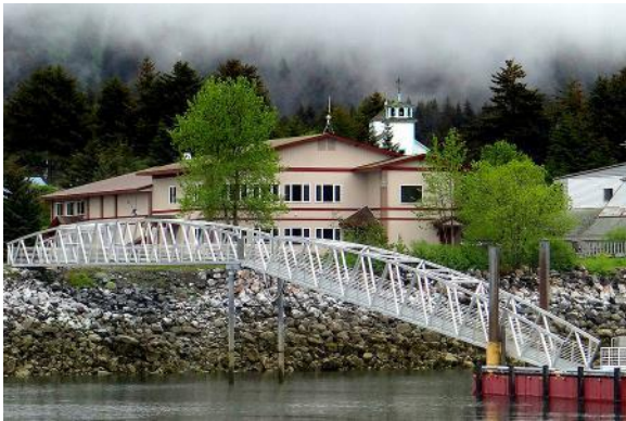
Ferry Dock Refurbishment
