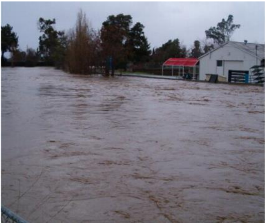
San Francisco Bay Levee Overtopping
