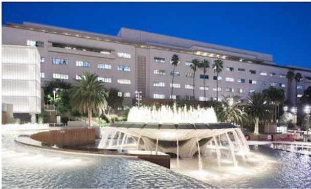
Government Building Seismic Retrofit
